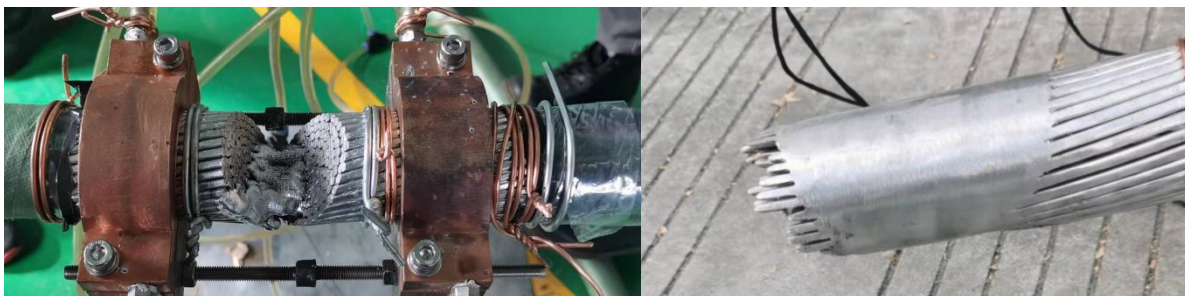
Figure 7 Aluminum conductor with joint V groove welded
