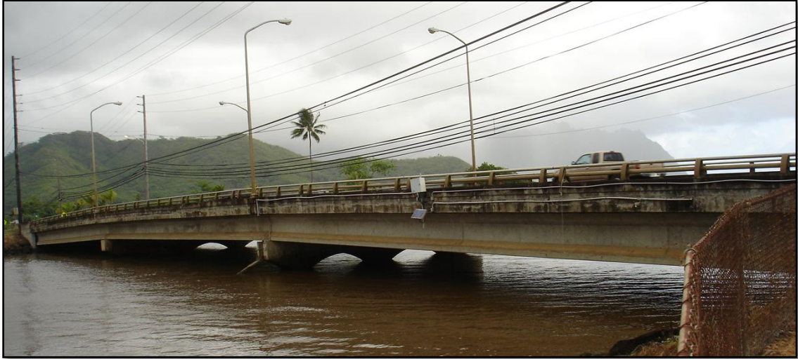
Figure 4-15: Photo of Kahaluu Bridge Looking East
