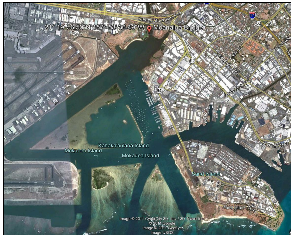
Figure 4-49: Moanalua Bridge Location
