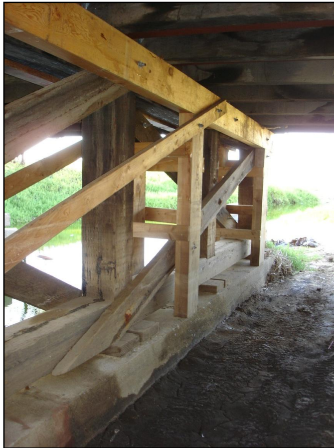
Figure 4-25: Wooden Bent
