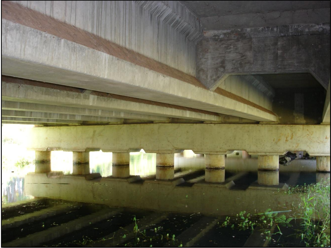
Figure 4-20: Photograph of Underside of Bridge Deck
