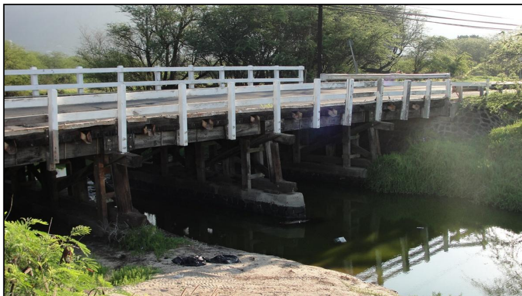
Figure 4-23: Photograph of Old Makaha #3A Bridge Looking South East
