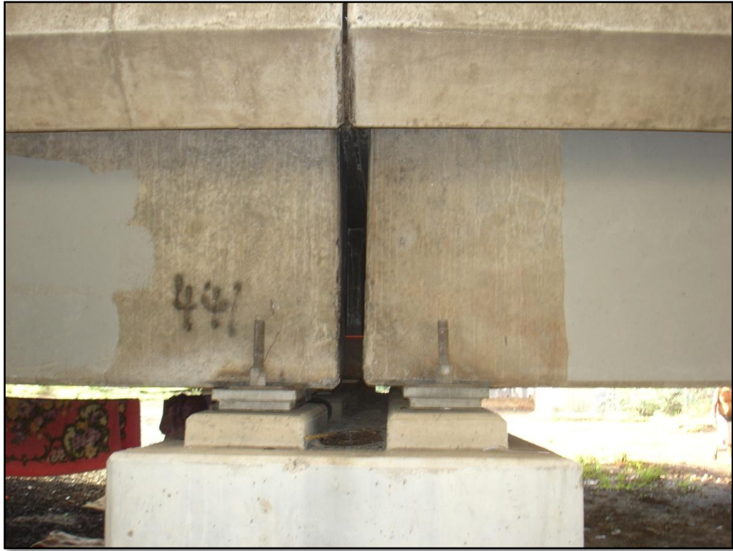
Figure 4-45: Moanalua Bridge Connections
