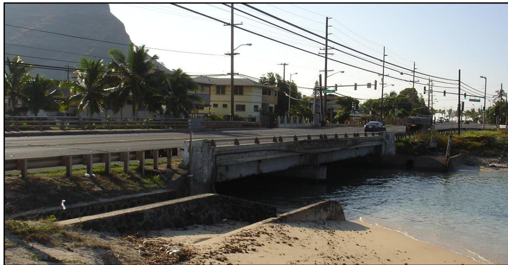
Figure 4-35: Photograph of Maipalaoa Bridge Looking South East
