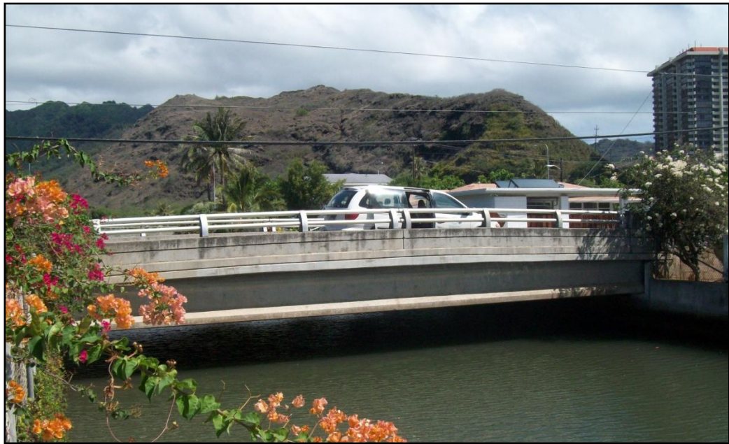
Figure 4-3: Picture of Kuliouou Stream Bridge looking north
