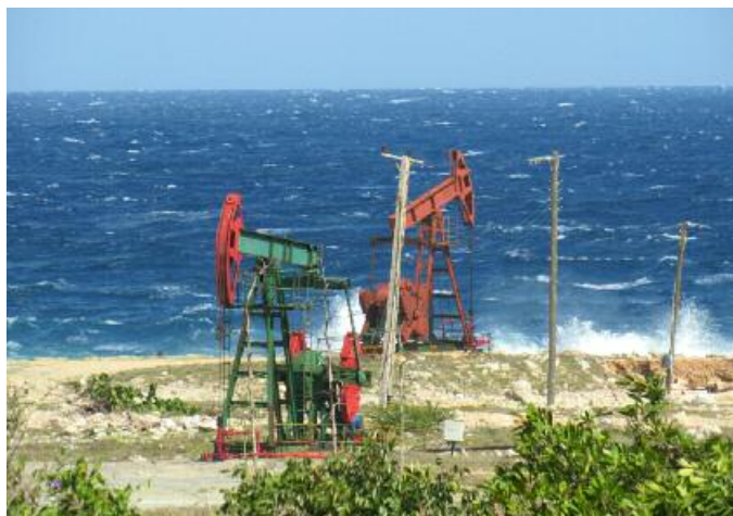
Figure 46. For the installation of the oil pumps, extensive areas of the coast are cleaned and cleared. After the machines are removed, invasive plants such as Yucca aloifolia L. are planted on some occasions, evidence of poor management of coastal recovery.
