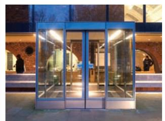
in the same brushed simulated stainless steel finish as the porch structure and two 130mm diameter stainless steel bollards with push pads have been installed to allow visitors to activate the doors. Pocket screens have been installed to ensure the safety of visitors to the gallery.
