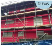
heavy-weight timber frame panels, with Wraptite-SA, self-adhering vapour permeable air barrier being applied on site. The use of Wraptite-SA makes a significant contribution to a building's thermal performance by preventing lateral air movement. It also provides high vapour permeability in a continuously sealed, self-adhered, airtight membrane.
