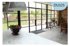
and installed by Steel Window Association member, Steel Window Service & Supplies. Three sets of double doors form the external screen which has an overall height of 3m and includes fixed lights above and between the doors. Measuring 2.4m wide x 2.6 high, the first of the internal screens divides the extension from the living room and is composed of double doors with fixed lights either side and above.
