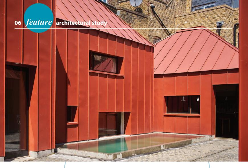
room. The roof-lights can be opened and, on warm days, the stack-effect ensures that fresh cool air is drawn in from above the pool. The Pantheon and the work of James Turrell have influenced the design of the top lit pavilions.
