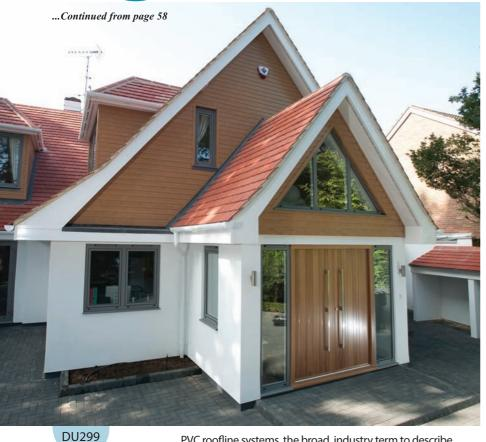
PVC roofline systems, the broad, industry term to describe fascias, soffits, bargeboards and all the associated ventilation components, are rather good at the double trick of protecting the eaves while fully venting them.
