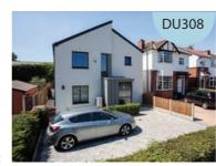
design. Architect, Sara Darwin, commented: "The Kingspan TEK Building System scored highly on thermal efficiency as the core insulation material has a lower thermal conductivity than other products. As a result, wall thicknesses could be minimised which was critical given the relatively tight plot. Minimising air leakage was also essential. A good airtightness result can reduce energy consumption by 1kwh/m²/a which can make all the difference between a pass and fail."
