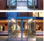
in the same brushed simulated stainless steel finish as the porch structure and two 130mm diameter stainless steel bollards with push pads have been installed to allow visitors to activate the doors. Pocket screens have been installed to ensure the safety of visitors to the gallery.
