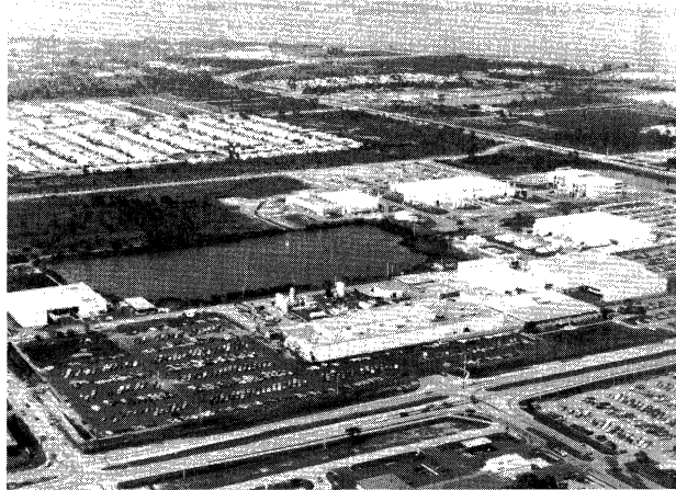
Harris Semiconductor's Melbourne, Florida, complex contains complete facilities for design, masking, wafer fab and final testing.
