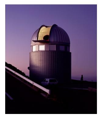
Figure 3.8: Photo showing the 1.2 m *Euler* Telescope, at La Silla, Chile. The échelle spectrograph CORALIE is connected at the Nasmyth focus via optical fibre. An imager is located at the secondary focus. Photo courtesy www.eso.org.
