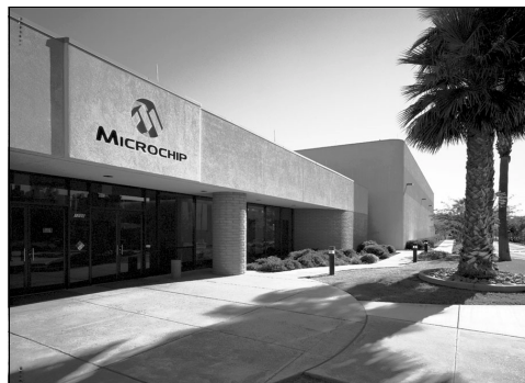
Tempe, Arizona: Microchip's 200,000-square-foot wafer fabrication facility provides increased manufacturing capacity today and for the future.
