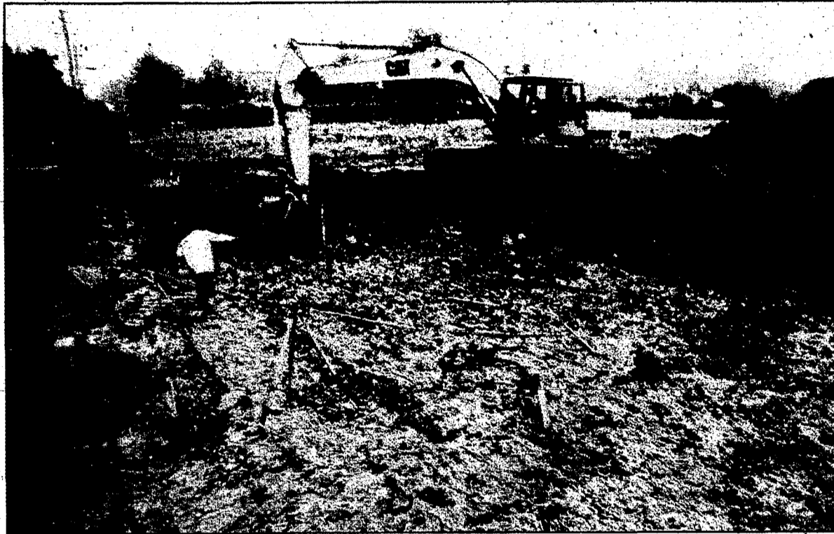
Work progresses: Excavators dig a basement at the Bayberry Park Subdivision in Livonia (left), while Ronald P. Benivegna and Alan M. Gottlieb, builders, look over plans in front of a model (below).
