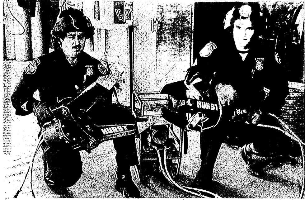
Equipment used for prying open a jammed car door to free a passenger and giant hydraulic compresser shears that can cut through
