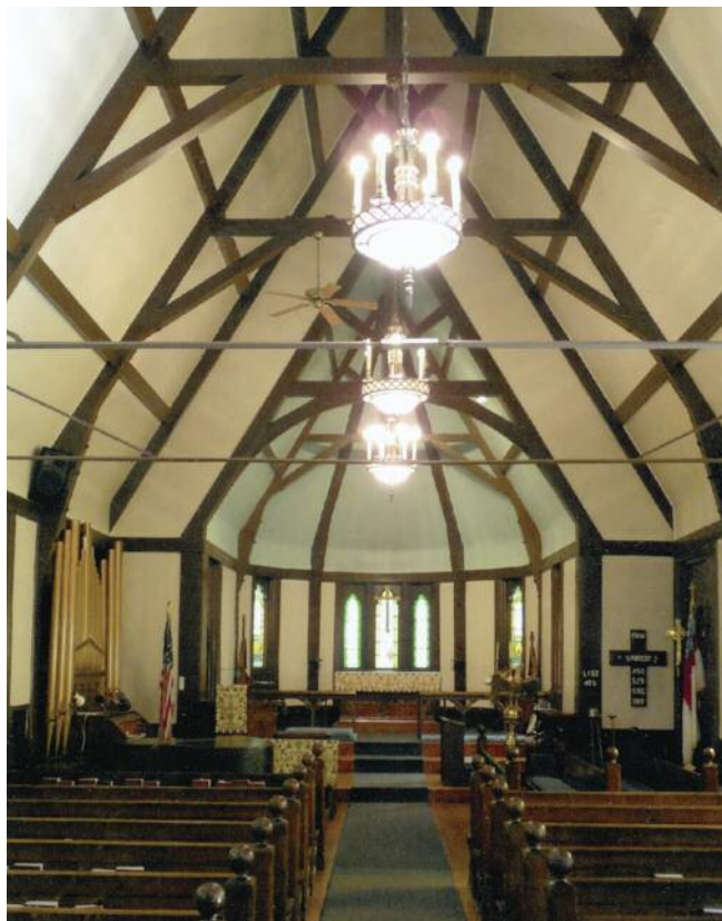
Top to bottom: Exterior of St. Mark's Episcopal Church, Ashland, New Hampshire. Courtesy St. Mark's Episcopal Church. Interior of St. Mark's Episcopal Church. The chandeliers and tie rods are later additions. Photo by James F. O'Gorman.
