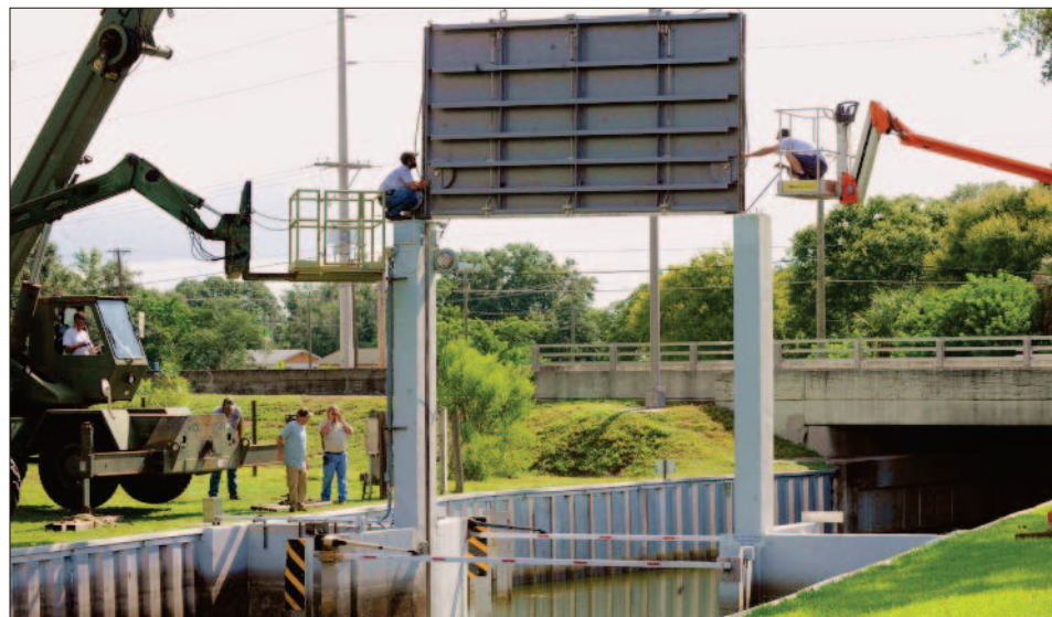
PHOTO BY CHARLES A BAKER III The “doors” in the “locks” connecting the North and South Chain of Lakes were repaired last week just in time for summer boating.
