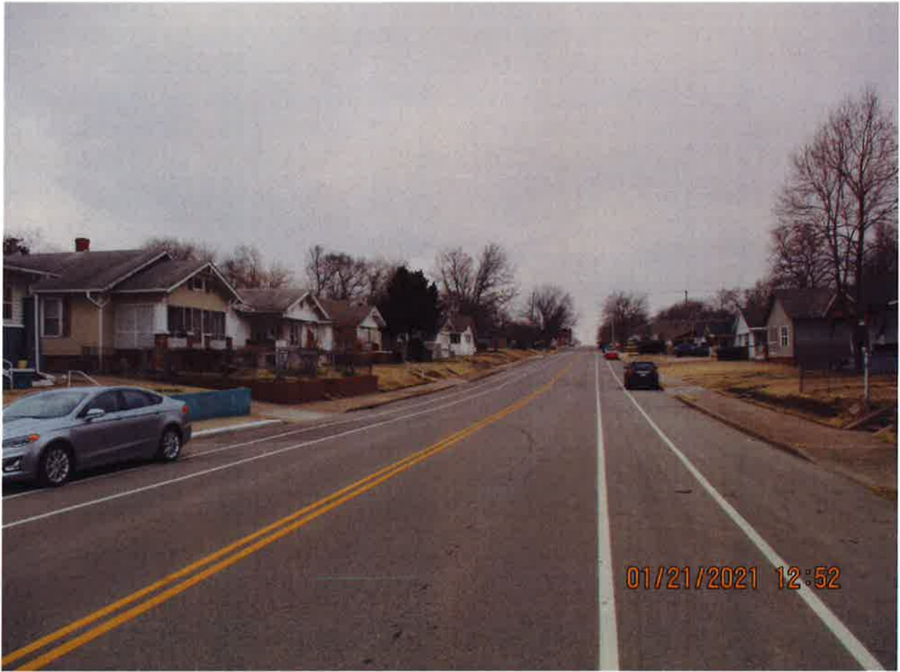
Facing North on Main
