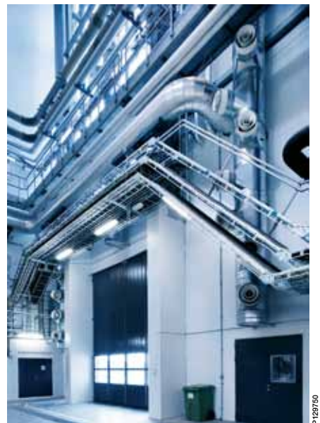
Wibe cable ladder KHZV installed at Gärdstaverken, Sweden.
