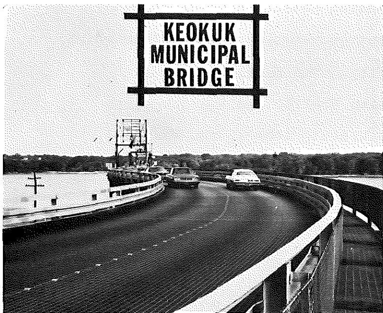
Reverse curve on Bridge at Iowa side.
