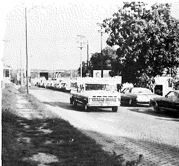
Traffic backed up from Municipal Bridge Tollgate.
