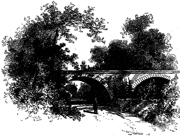
BRIDGE CONNECTING NORTH AND SOUTH LAUREL HILL.
