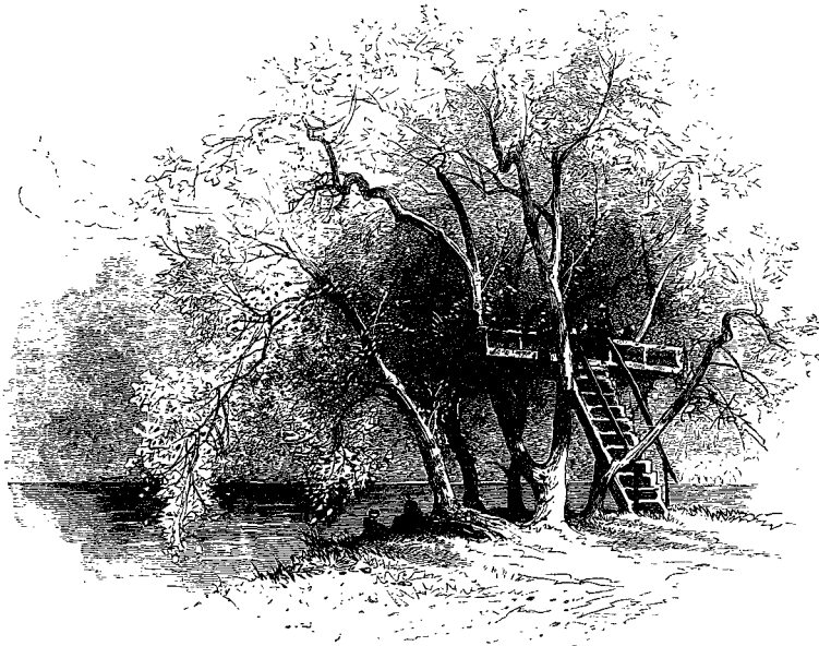
PLATFORM IN TREE.
