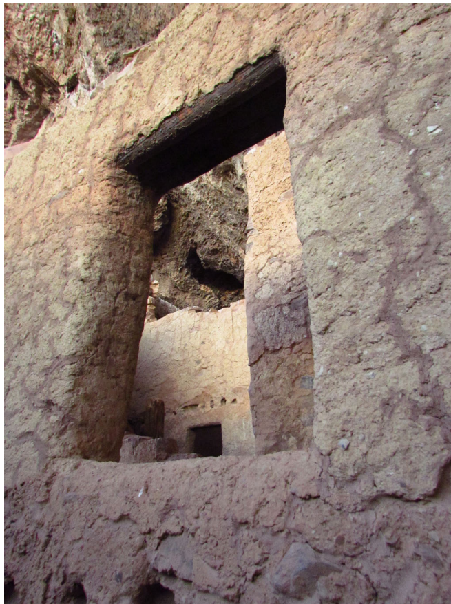
Figure 11. Photograph of adobe-covered walls in the Upper Cliff Dwelling. Construction began about 1300 CE and continued until between about 1400 CE and 1450 CE. The size of the cave, with 24-m- (80-ft-) high ceilings, allowed for living quarters with second and third story rooms. NPS photograph by C. Sadler (Tonto National Monument) available at https://www.flickr.com/photos/tontonps/ (accessed 12 June 2019).
