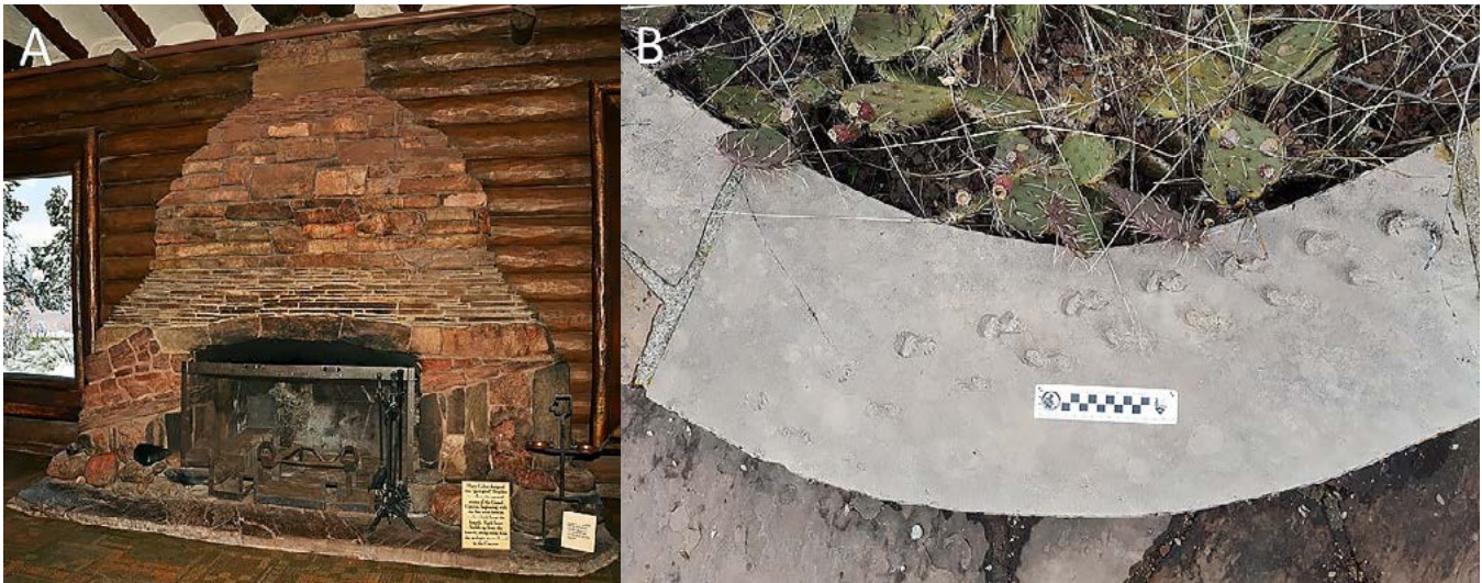
Figure 18. A. The geology fireplace in the Bright Angel Lodge designed by Mary Colter exhibits geology and paleontology of the Grand Canyon (NPS/MICHAEL QUINN). B. Fossil trackway slab used as building material for a bench in the Grand Canyon Headquarters courtyard. (NPS/DIANA BOUDREAU).
