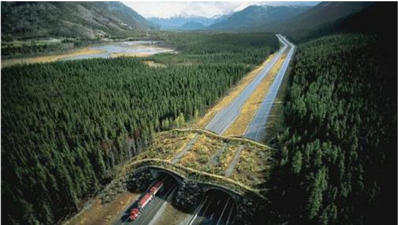
Overpasses to create ecosystem connectivity and reduce human wildlife conflicts (collisions) © Parks Canada
