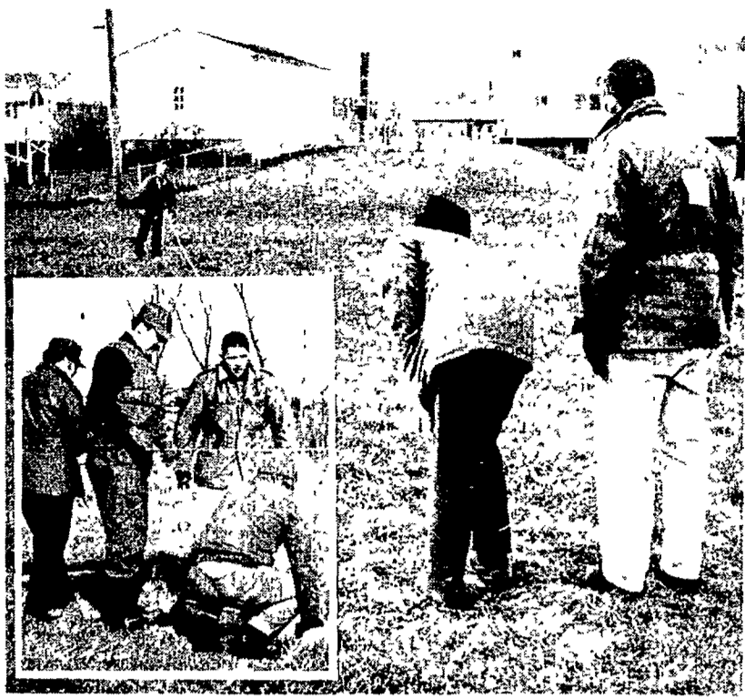
RINK MAKERS — Northville Jaycees, who joined with Recreation Director Robert Prom in preparing sites for several ice rinks Saturday, had their fingers crossed in hopes of freezing weather this week. Rinks are planned at Ford Field, Village Green Subdivision, and at several other locations. Meanwhile efforts are being made to secure materials and volunteers for construction of small rink shelters. Interested persons are asked to call John Buckland at 349-0773 or Cecil Morin at 349-5707.
