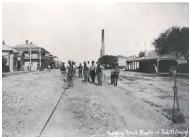
Laying ‘the steel track’ in Edith Street, circa 1906. The Edithburgh Hotel is on the left.
