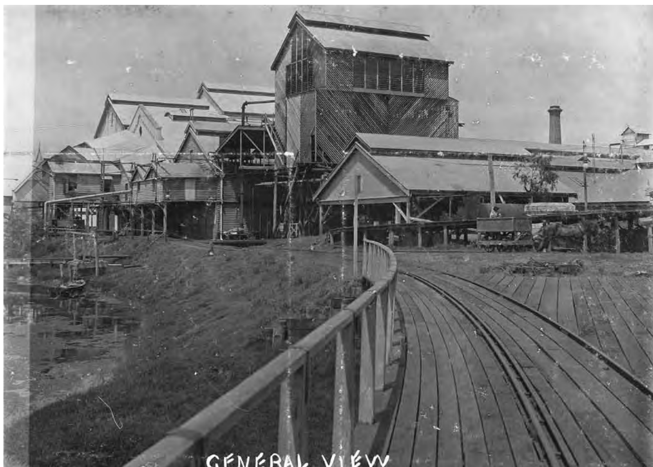
On wharves and bridges, decking was provided for the horses. This appears to show the track coming off the bridge that crossed Lakes Creek, complete with checkrail. In the background can be seen a horse hauling a tip truck with a rectangular body. Photo: State Library of Queensland 126583
