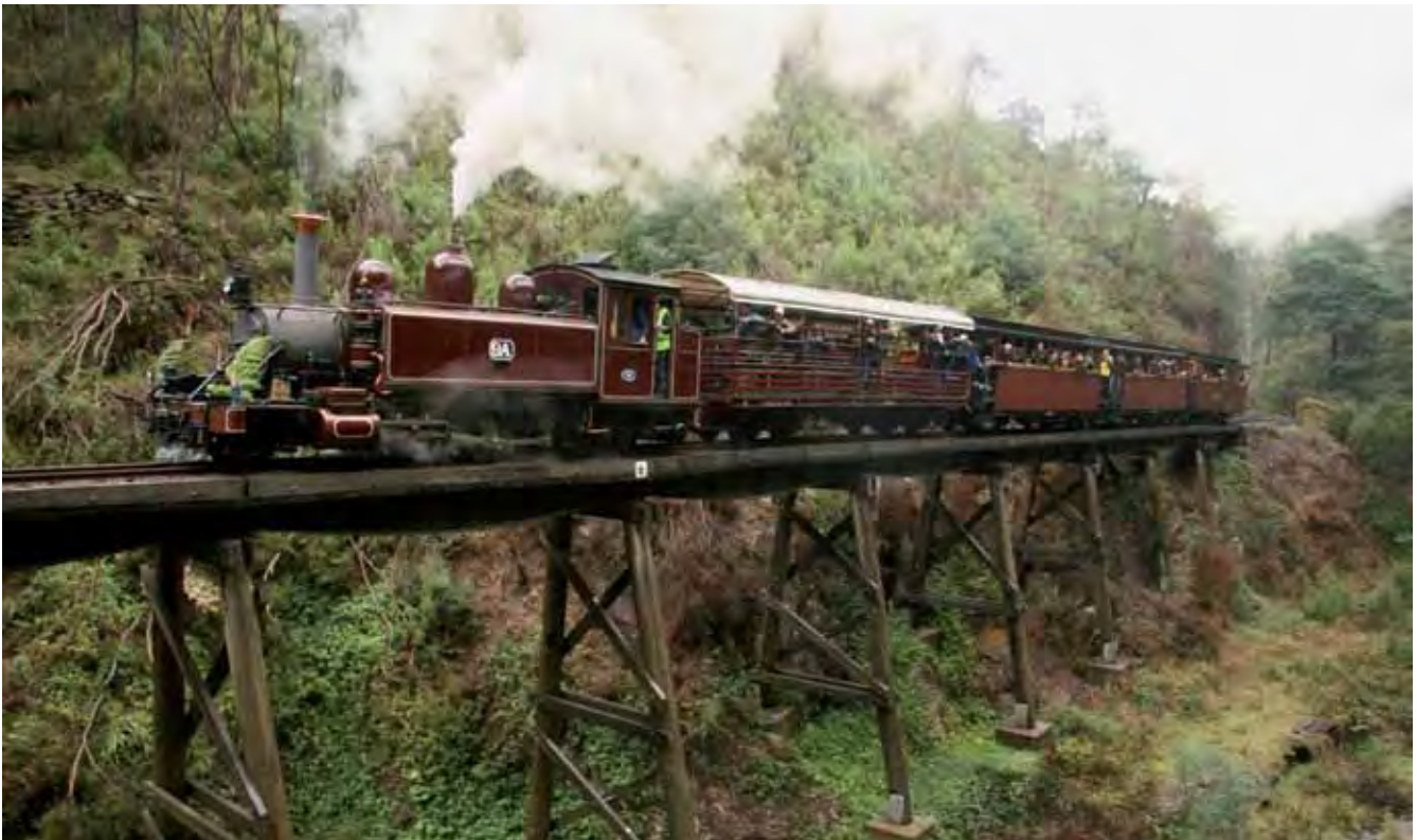
'9A' crossing one of many trestle bridges in Stringers Gorge on Saturday 29 May. Pounding up the 1 in 30 grades, the sound reverberated spectacularly off the canyon walls. Photo: Nick Anchen
