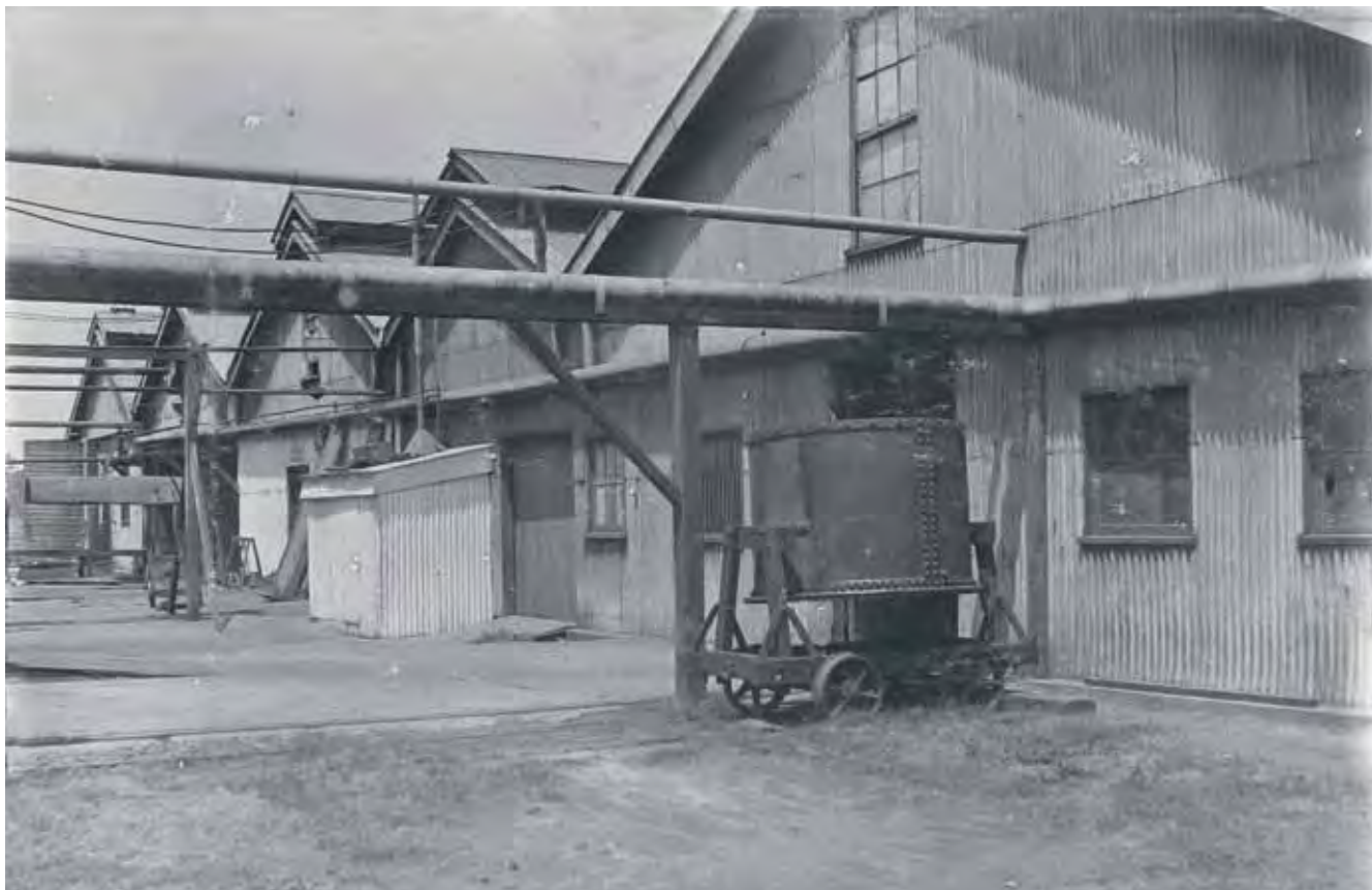
An interesting tip wagon. It has timber framing with iron bracing and inside journals. Buffer beams and new couplers were added to the rolling stock when the Lister locomotive arrived.
