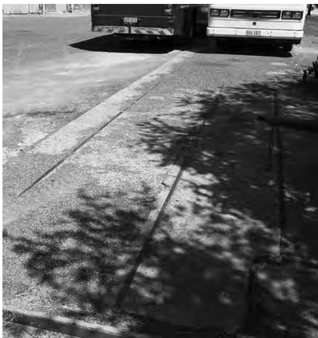
Remains of the tramway that ran within the box shed set in concrete at the western end of the site in January 2007. Photo: Author
