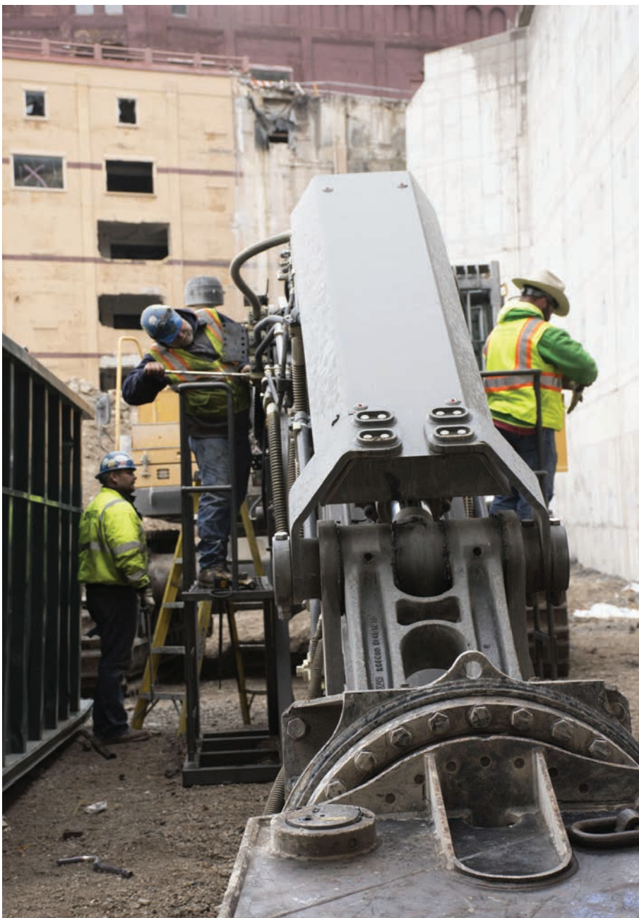
An innovative design makes it easy for the crew members to change the boom quickly and efficiently.
