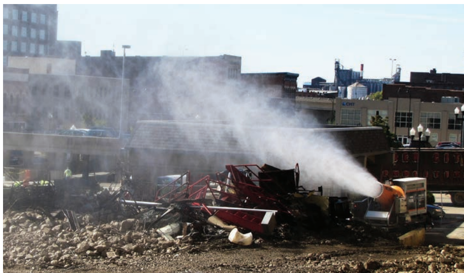
The atomized misting unit can deliver up to 62,800 sq. ft. (5,834 sq. meters) of coverage.
