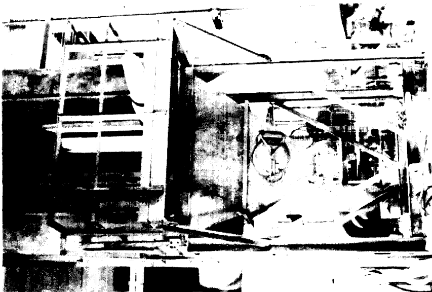
FIGURE 8 THE BNPDS RADIOACTIVE WASTE INCINERATOR EXHAUST GAS FILTER BAG-HOUSE
