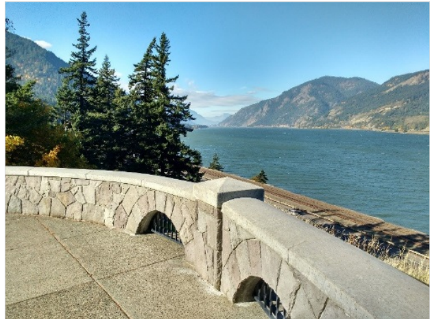
Figure 1: View of the Columbia River Gorge from the HCRH State Trail
