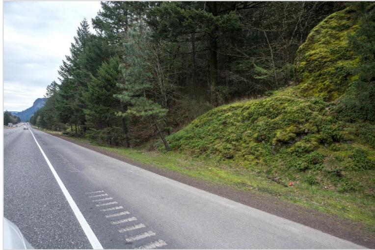
Figure 10: Existing View I-84 Eastbound at Ridge Cut
