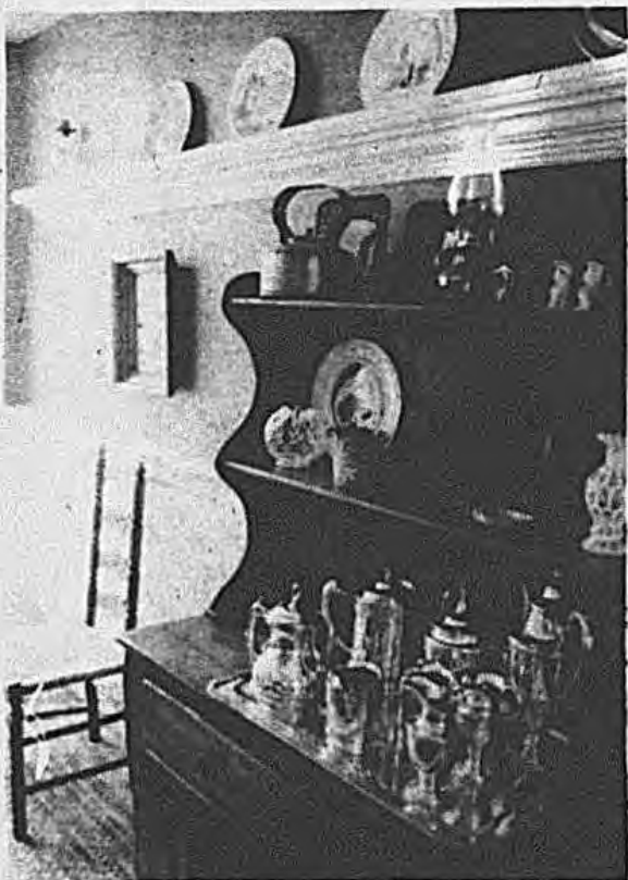
TRADITIONAL TOUCH — Ready-made moldings can be used in new construction to re-create the plate rails, dados and chair rails typical of older traditional housing. Design by Marc Tarasuck.
