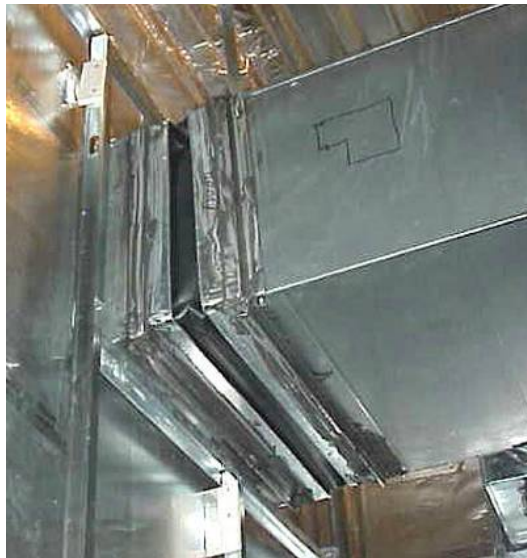
Figure 3-6 Duct Penetrations
