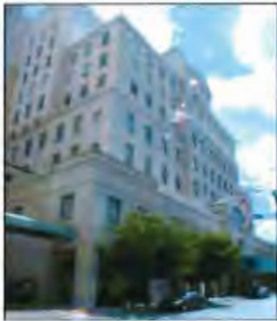
Appropriate: a stepback is provided at 30 feet, the predominant height along the block. Additional stepbacks are provided as the building increases in height.
