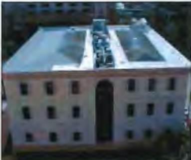
Appropriate: utilities are centrally located on the roof.
