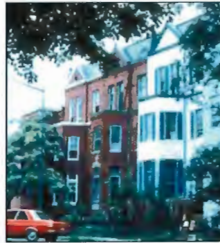
Inappropriate: the townhome on the right has had its original brick facade covered by vinyl siding.
