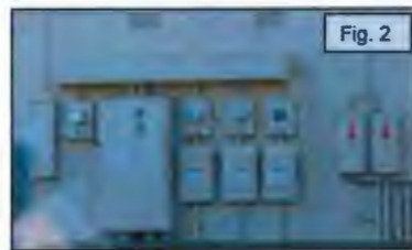
Appropriate: utilities such as gutters, downspouts (fig. 1) and utility boxes (fig. 2) have been painted to match the primary building color.
