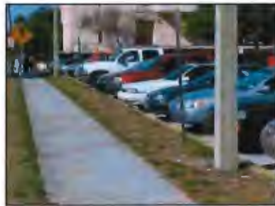
Inappropriate: parking lot is unscreened and cars are parked directly along the right-of-way.
