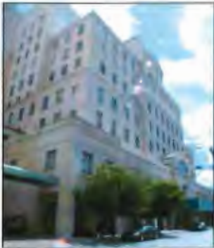
Appropriate: a stepback is provided at 30 feet, the predominant height along the block. Additional stepbacks are provided as the building increases in height.
