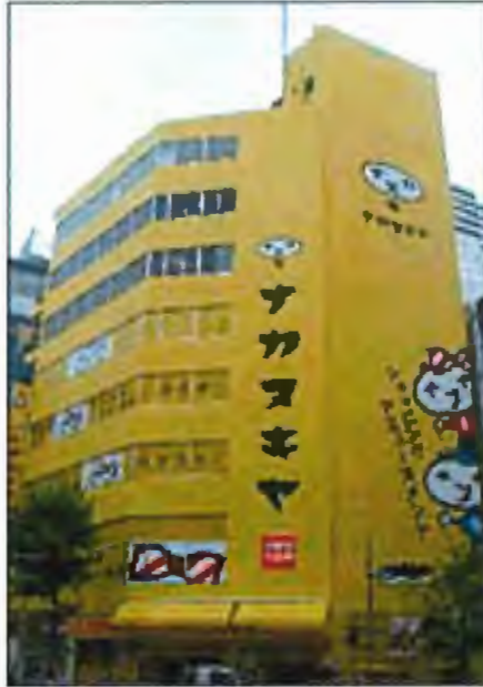
Inappropriate: loud and garish colors.
