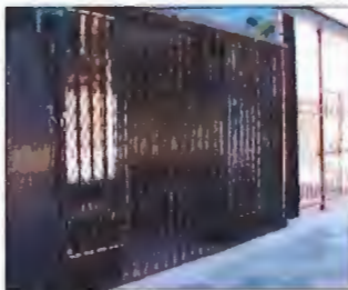
Inappropriate: security gates
