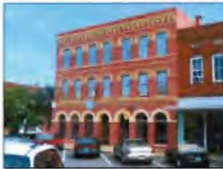
Appropriate: the raised banding provides rich detail and differentiates the various floors.
