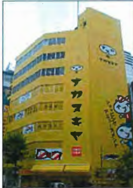
Inappropriate: loud and garish colors.
