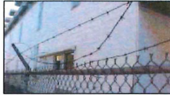
Inappropriate: chain link fence and barbed wire.
