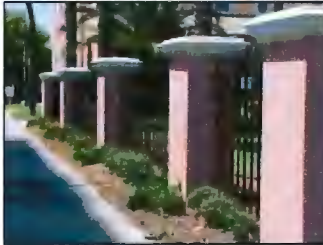
Appropriate: fence with masonry columns matches the color and materials of the principle structure.
