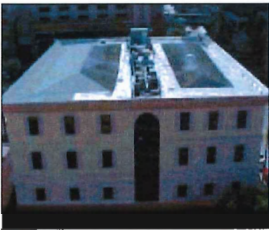
Appropriate: utilities are centrally located on the roof.
