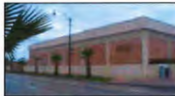
Inappropriate: this building does not include windows along the street.
