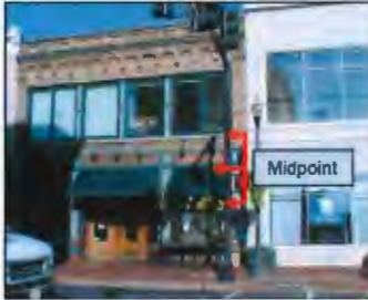
Appropriate: awning is correctly located on the façade of the building.
