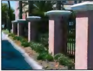
Appropriate: fence with masonry columns matches the color and materials of the principle structure.
