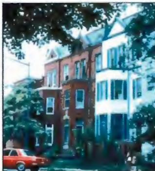
Inappropriate: the townhome on the right has had its original brick facade covered by vinyl siding.
