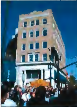
Appropriate: this building has a very distinct base, middle and an understated cap
