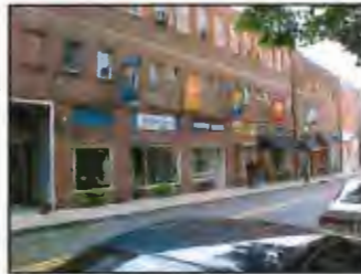
Inappropriate: façade extends over 50 feet without detail or articulation.
