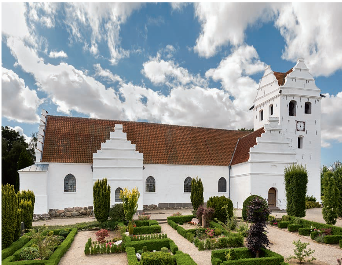
Fig. 10. Kirken set fra nord. Foto Arnold Mikkelsen 2016. – The church seen from the north.
