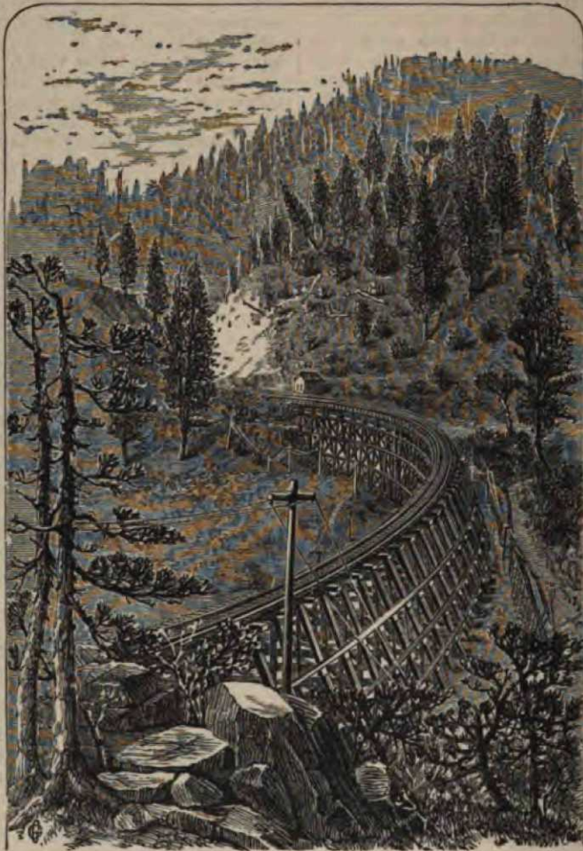
SECRET TOWN, TRESTLE-WORK.
