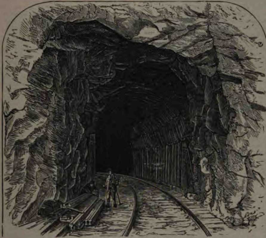
TUNNEL NO. 12, STRONG'S CANON.
