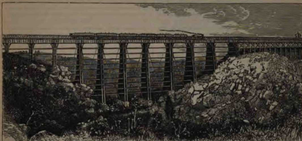
DALE CREEK BRIDGE.
