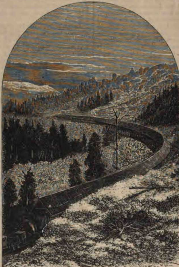
SNOW SHEDS ACROSS THE SIERRAS.
