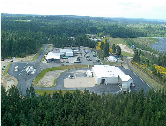
Olympic View Transfer Station
