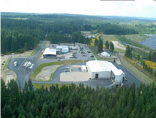
Olympic View Transfer Station
