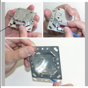
6 Place the Housing inside the Jack hole. Trim wall cutout if necessary.
