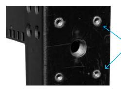
Optional Caster mounting point, on bottom of rack frame
