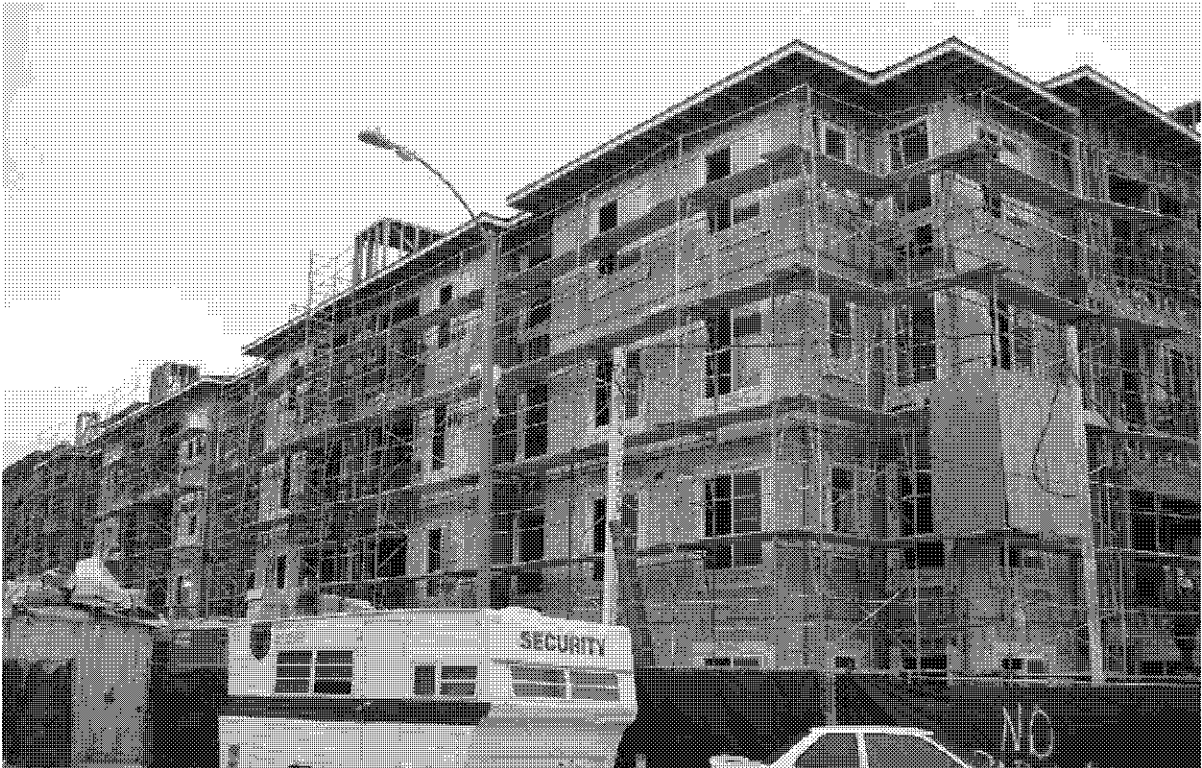
Rear of subject northwest corner
