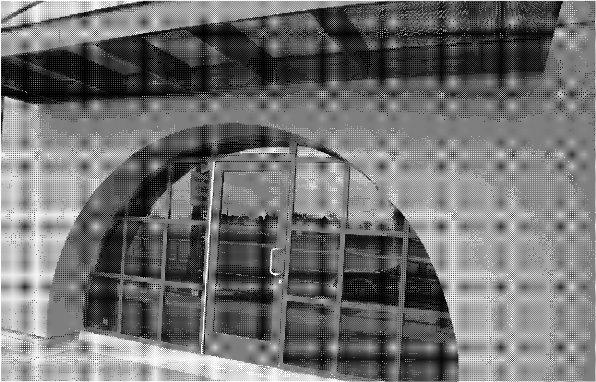
Retail Unit #1005, Subway space
