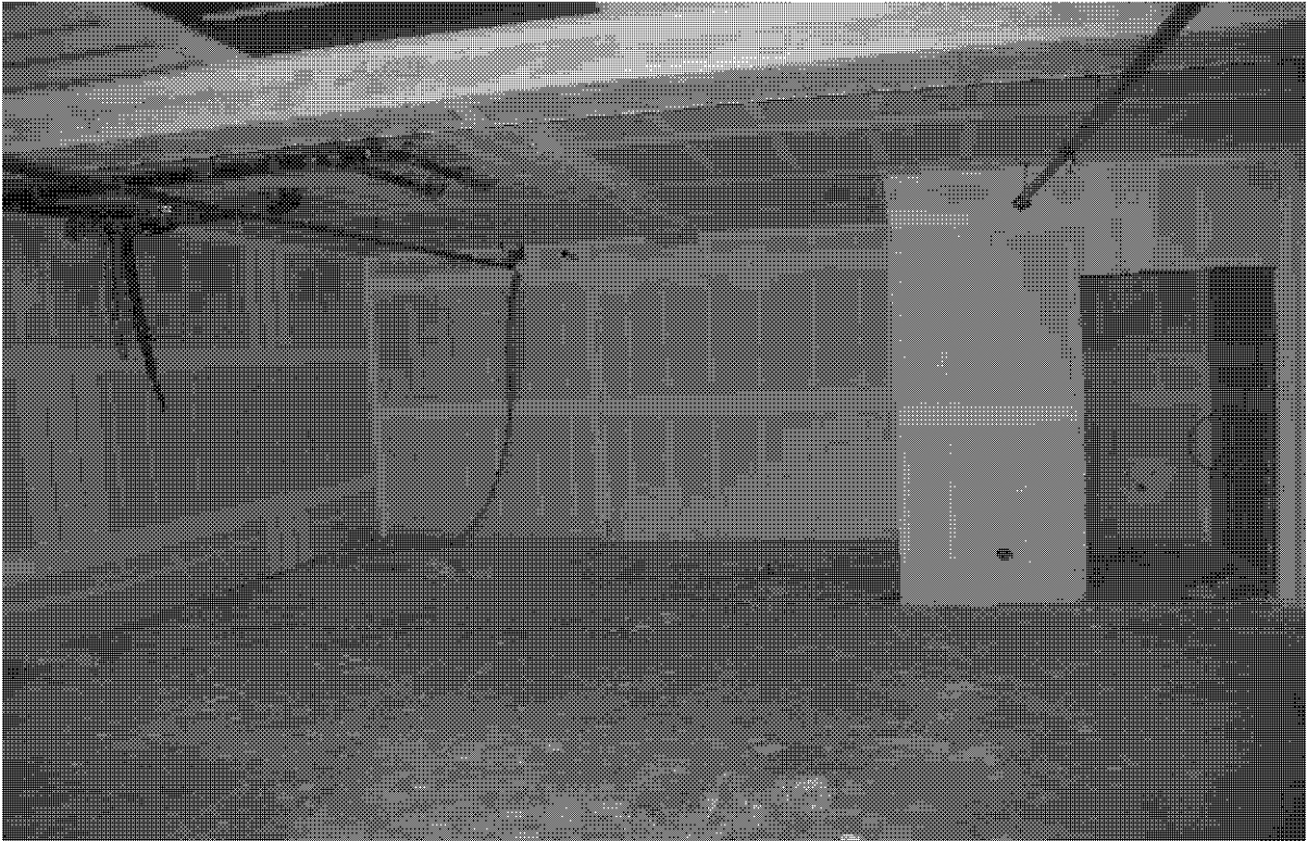
Interior of Retail Unit #1005, Subway
