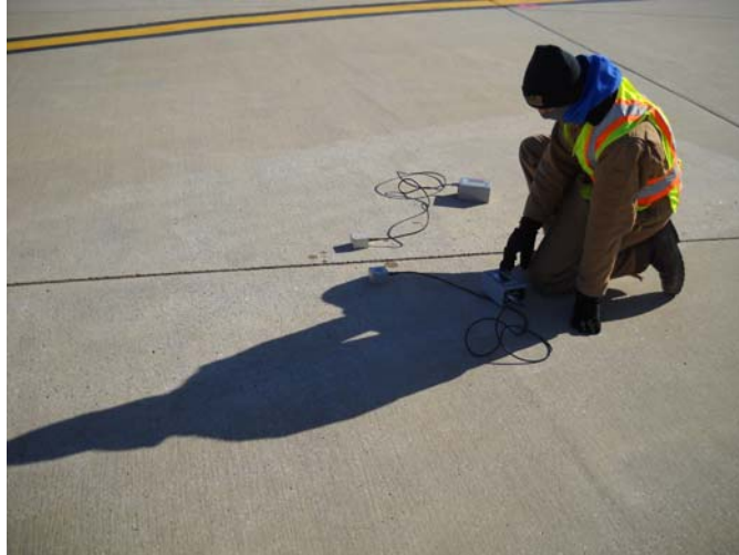
FIGURE 3.43. SLAB ROCKING TEST IN PROGRESS.
