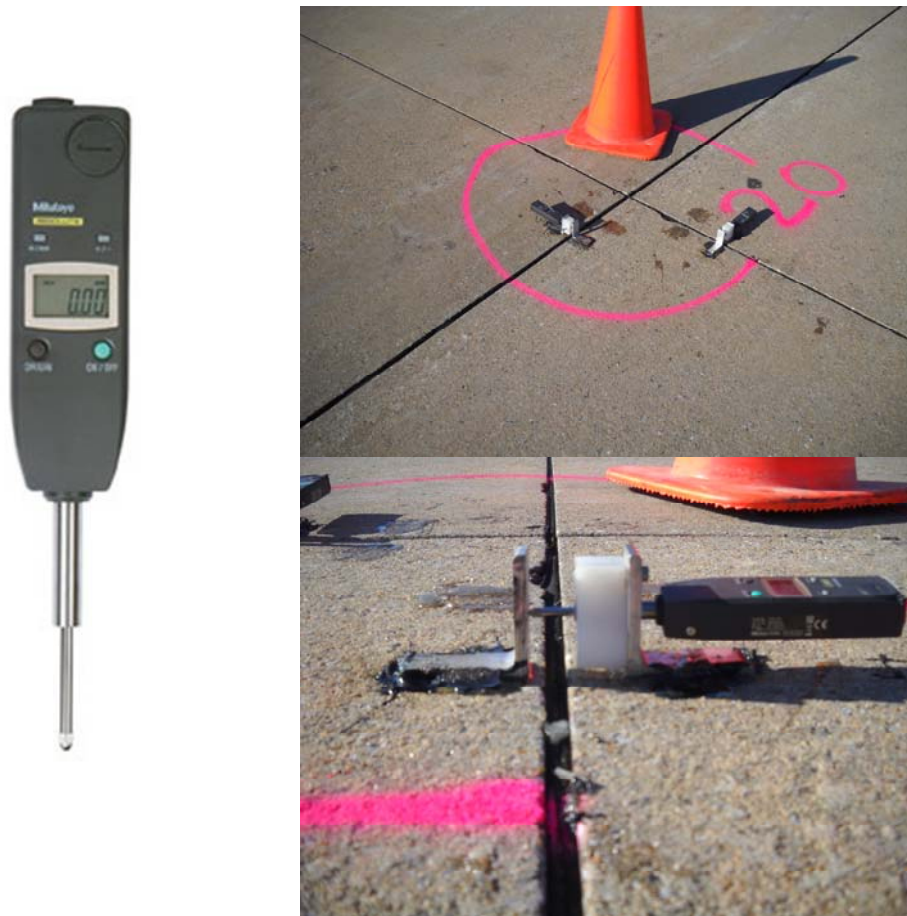
FIGURE 3.38. MITUTOYO DIGITAL INDICATORS USED TO MEASURE THE CHANGES IN JOINT OPENING SIZE
