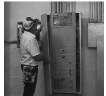
The three-piece trim for larger power distribution panelboards provides for easy handling and installation
