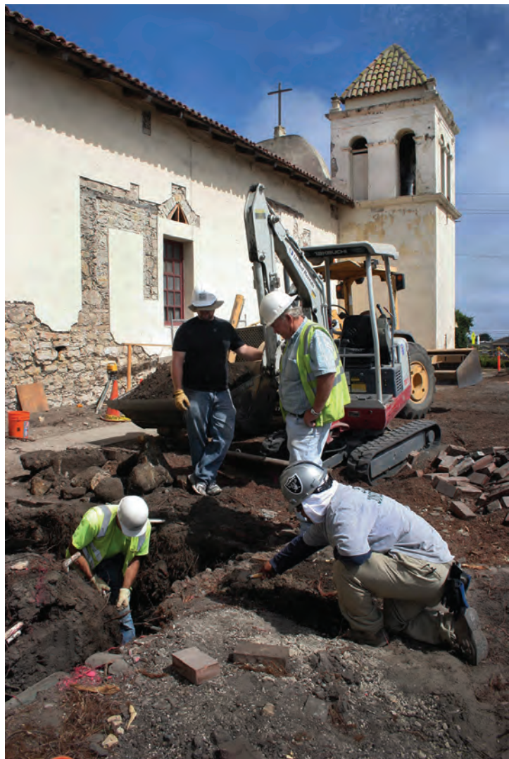
Figure 3. In order to mitigate against the continued deterioration of the shale and mudstone due to water intrusion and salt erosion, the Royal Presidio Conservation Project of the Diocese of Monterey undertook the large-scale installation of a French drain system. In order to see through this process, fourteen 22-foot to 25-foot long and 18-inch wide trenches were excavated to bedrock along the entirety of the perimeter of the Royal Presidio Chapel (aka: San Carlos Cathedral). Photo © Rubén G. Mendoza, 2007.
