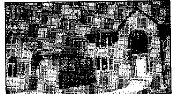
HOWELL. New community. Howell's newest sub, towering trees w/serene setting. 2 story Tudor home has 4 BR, 2 1/2 lavs, 3 car garage. Full bsmt, spacious gourmet kitchen, library, family room. Howell schools. $499,999 (31HIG) 248-626-8800
