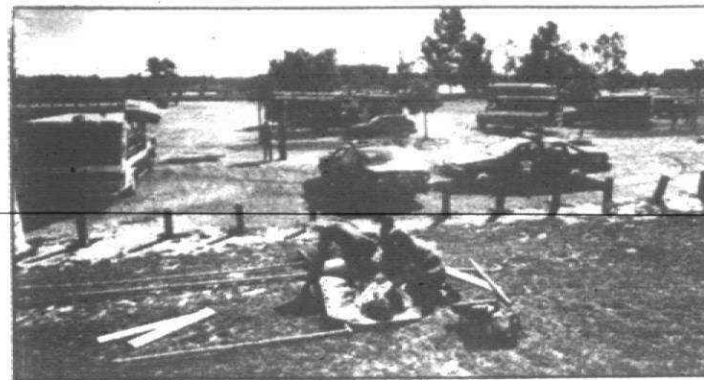
Scene of the mock tornado.
