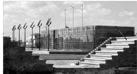
Figure 5. Greensburg's new identity via LEED buildings replacing conventional buildings
