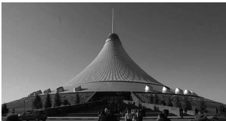
Figure 2: Khan Shatyr Entertainment Center, designed by Foster + Partners. Source: Flickr user Ken and Nyetta, 2011
