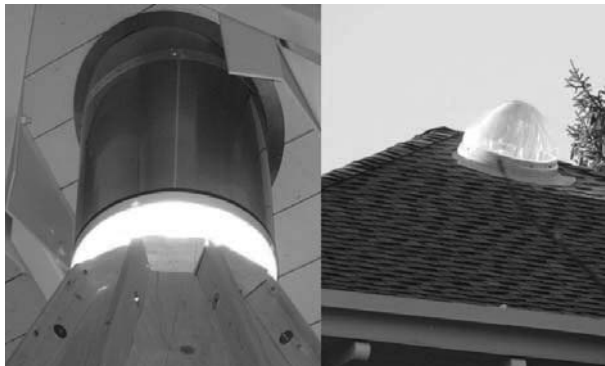
Figure 1: Skylight mounting details, interior and exterior.
