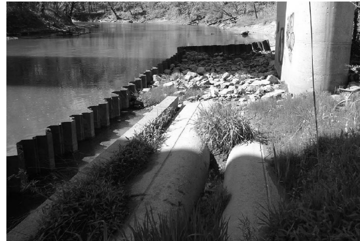
VIEW SOUTH FROM PIER 2; SN 092-0007 WB
