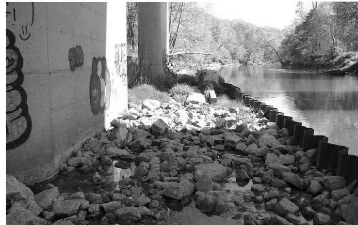
VIEW NORTH FROM PIER 2; SN 092-0006 EB
