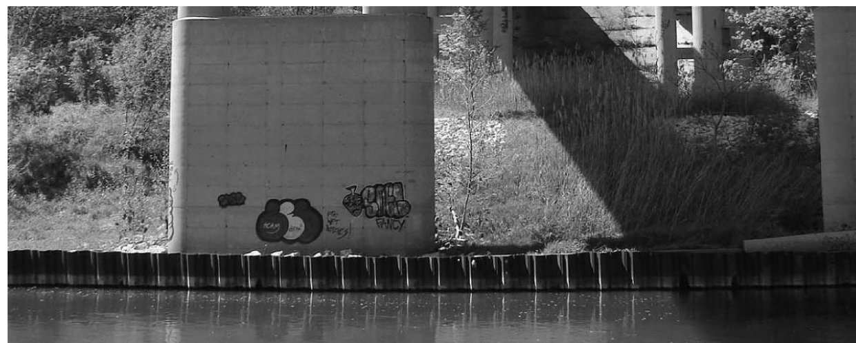
VIEW WEST AT EAST FACE OF PIER 2; SN 092-0006 EB
