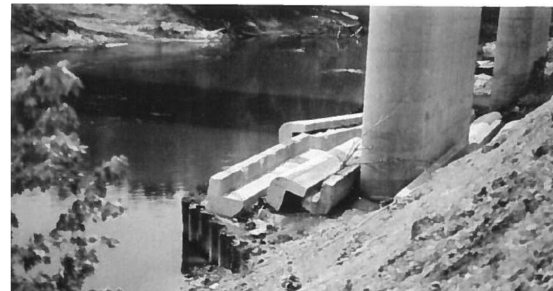
VIEW AT NORTH END OF PIER 2; SN 092-0007 WB
